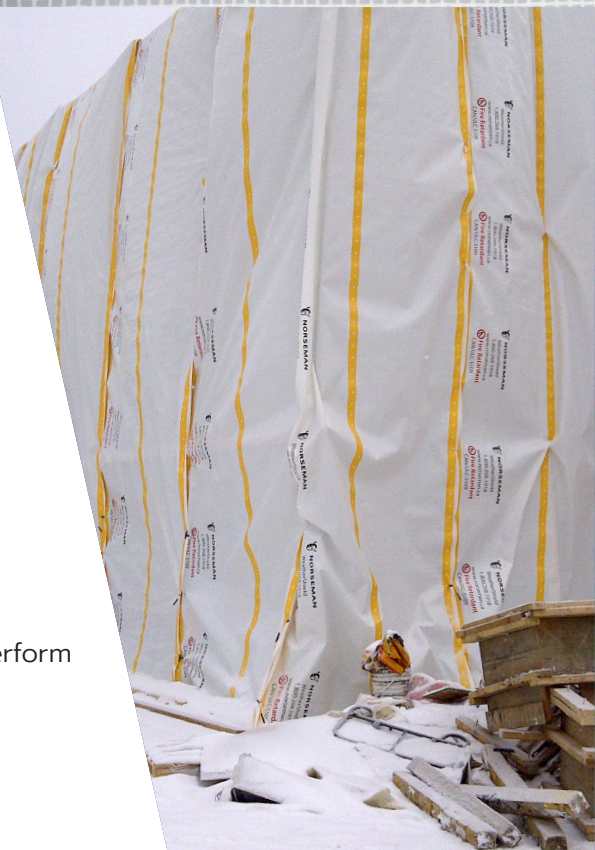
Manufactured with scrim-reinforced polyethylene material.
