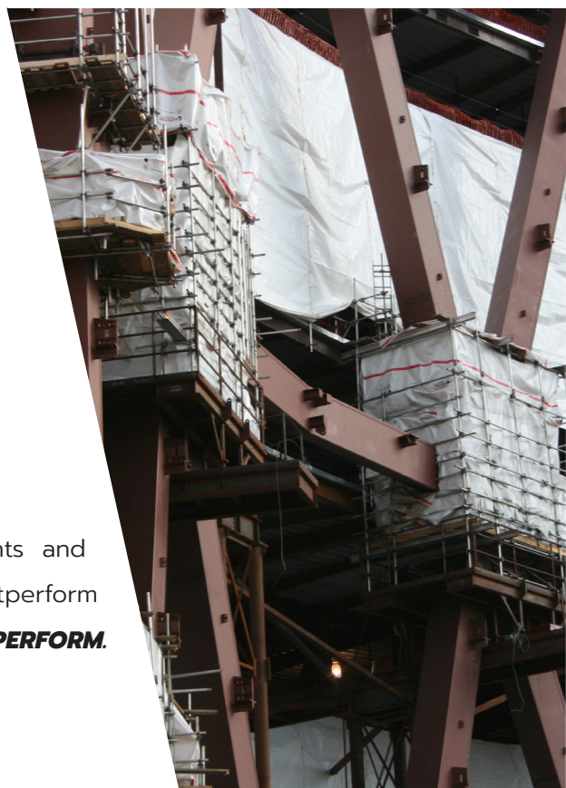
Sturdy 6.0 oz. polyethylene material with interlocking design.
